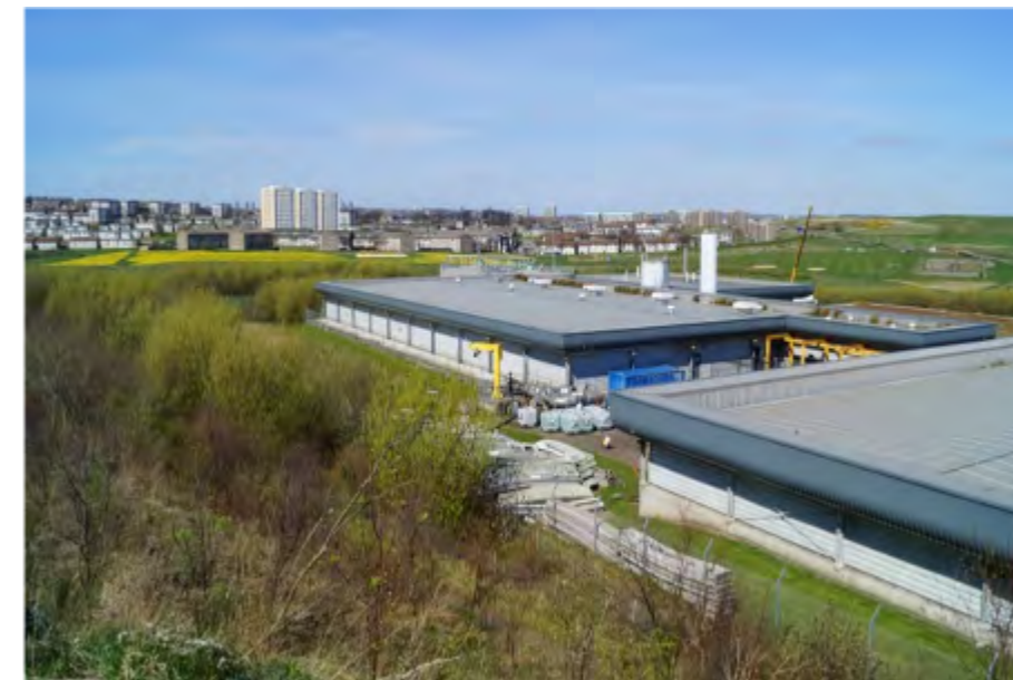
Nigg Waste Water Treatment Works
